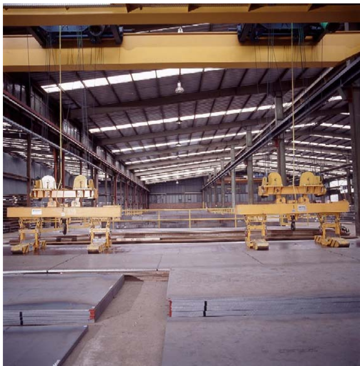
Fig. 5: Storage yard of Salzgitter Trading at its Gladbeck site
