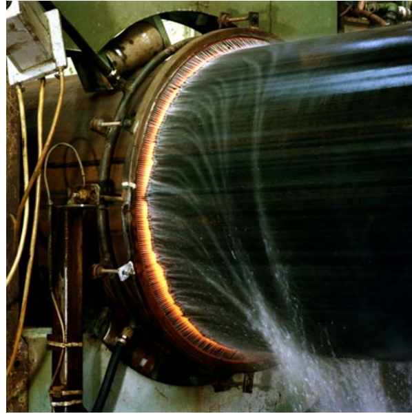
Figure 9: Detailed view on induction coil and heated zone during bending
